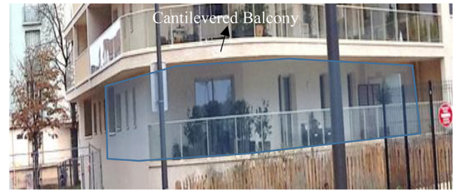
Fig. 5. Real image of the concerning building at upper ground.
