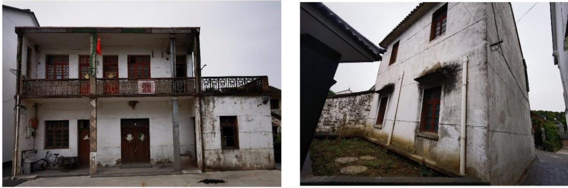
Fig. 5. Residential masonry building before renovation.
